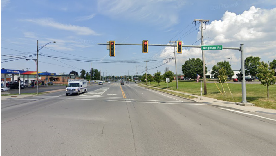
Example of traffic signal with high-visibility back plates and pedestrian signal equipment
