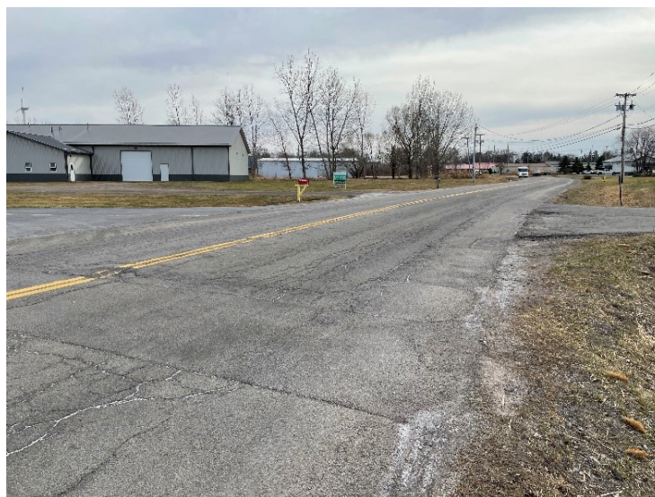
Existing pavement condition along Dean Parkway
