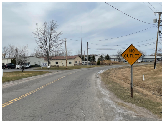
Typical roadside swale along Dean Parkway
