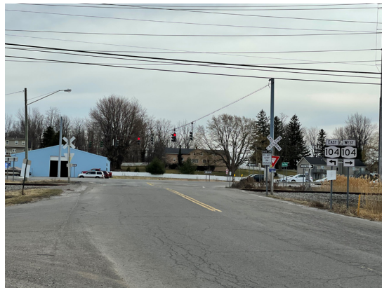
Dean Pkwy & NYS Route 104 intersection signage
